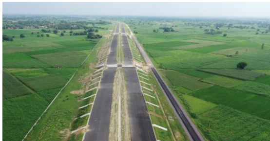
ARTL (Ganga Expressway)
