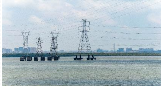
AESL (Mumbai – Vikhroli Transmission Line)
