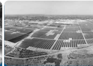
648 MW Ultra Mega Solar Power Plant
